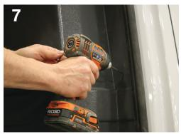
Loosely attach the partition with the 1  $\frac{1}{2}$ " Philip screws (**D**), flat washers (**B**), and split washers (**C**) to all areas where plus nuts were installed in step 5.
